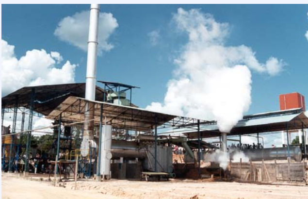
Palm oil processing plant in Neshuya, Peru
